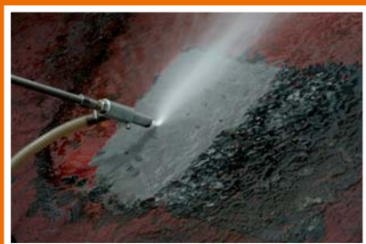
Surface - Sand Blasting
