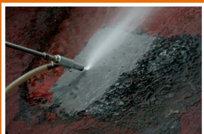
Surface - Sand blasting
