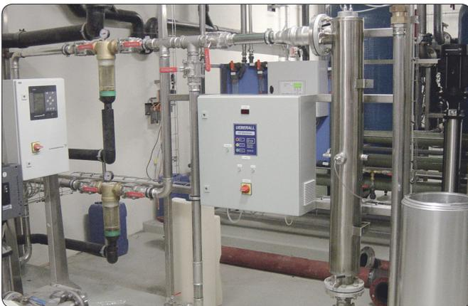
*At the Nestlé „Nespresso“ production site in Avanche, Switzerland, 3 units UB2-2 disinfect 25 m<sup>3</sup>/h each of filtered rain water and helps to save potable water for toilet flushing and on site cleaning every day*
