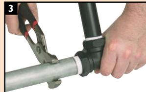
**3.** Do not over tighten. The right way to assemble a Threaded Pipe Fitting is finger tight plus one to two turns - no more!
