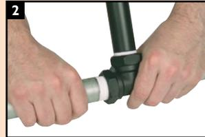
**2.** Screw pipe into fitting.
