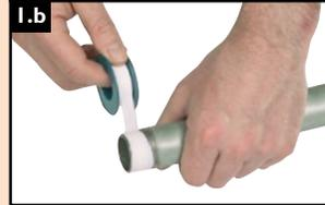
**1.b** Use a teflon tape sealant. The right sealant for threaded joints is non-hardening, compatible with plastic and doesn't add slipperiness to encourage over-torquing.
