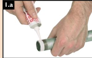
**1.a** Use a threaded paste sealant, we recommend LOCTITE 5331 or.....
