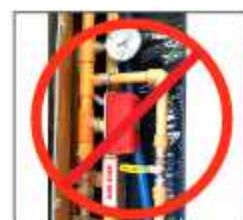
INCORRECT (No pressure relief valve)
