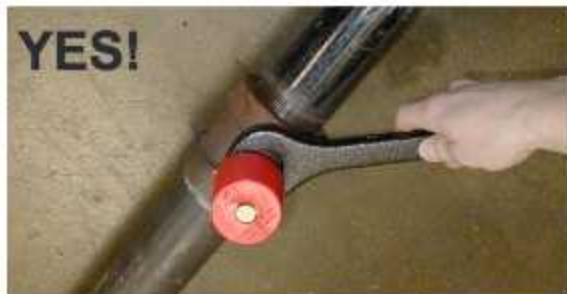
Figure 1: Correct use of designated installation wrench with ESFR Pendent K14 Sprinkler SIN VK500 and sprinkler cap
